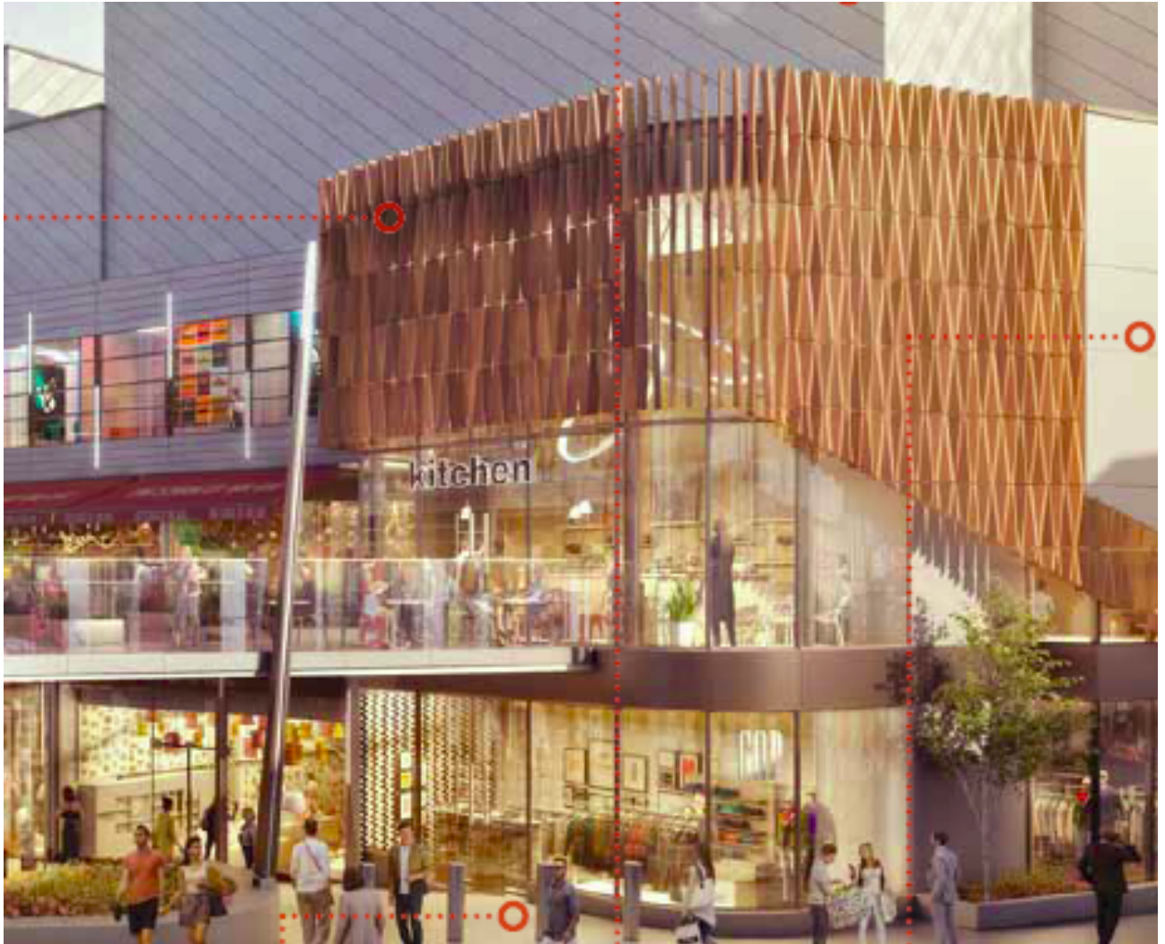
Figure 10.8 Detailed Render of proposed terracotta cladding
