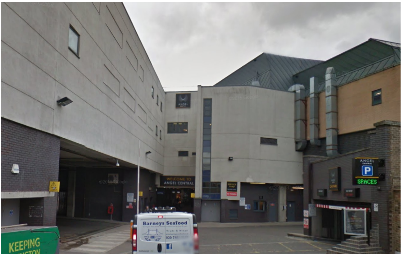
Figure 5.7 Parkfield Street Entrance, with car park entrance and servicing bays.
